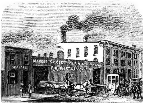
VIEW ON MARKET STREET, BETWEEN 15TH AND 16TH STREETS.
